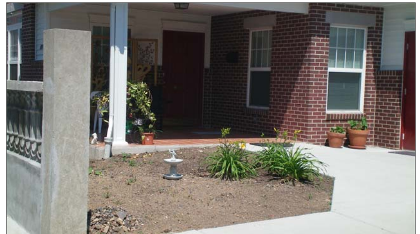
An example of one of the Pradera II housing units, a project developed by Asociación Puertorriqueños en Marcha (APM) in which all 53 units are Visitable.
