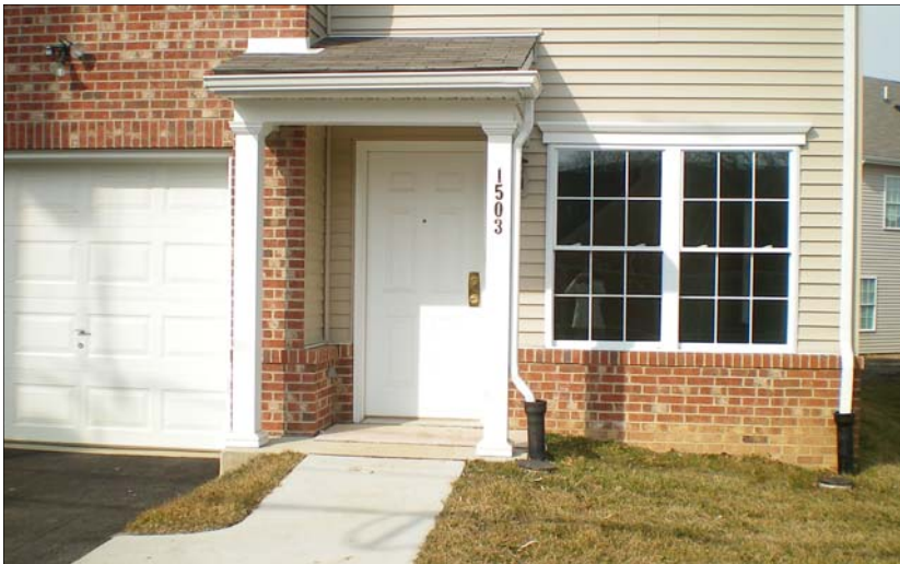
Visitable entranceway at one of the units at The Twins at Powder Mills .
